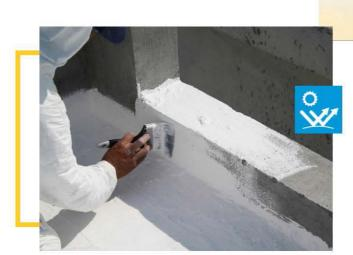
Provides sandwich membrane for Sunken Area, Roof, Terrace as well as Basement
